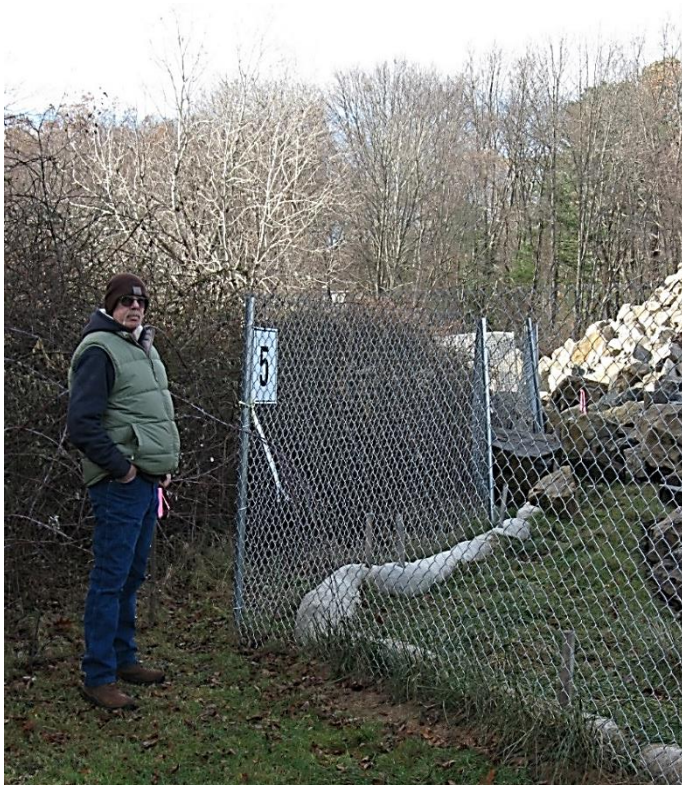
Paul Lewis at his property boundary, 11/25/17. Boulders have broken the construction fence and tumbled onto his property. According to the Construction Mitigation Plan, this area should not have been used for stockpiling excavated material.
